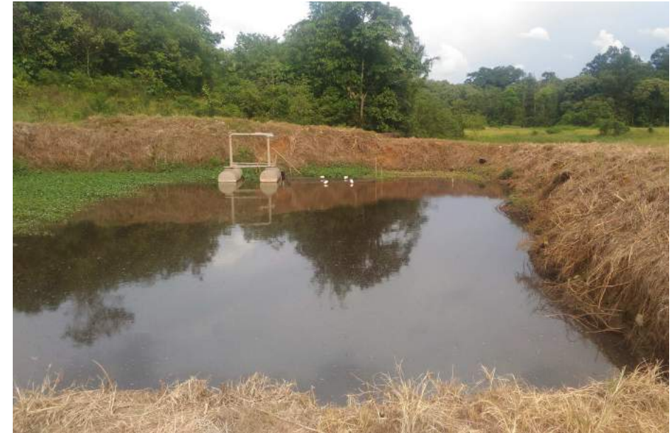
Palm factory waste management field
