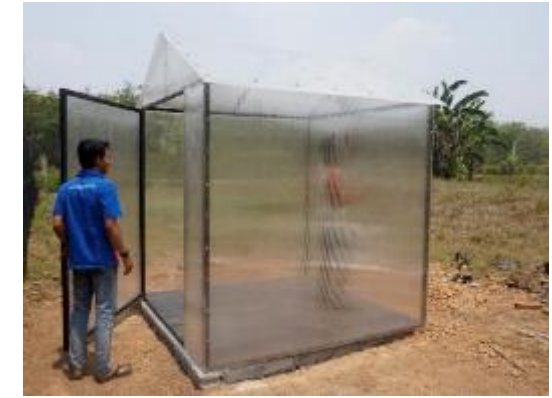
3 Placement of the solar dryer frame on the foundation
