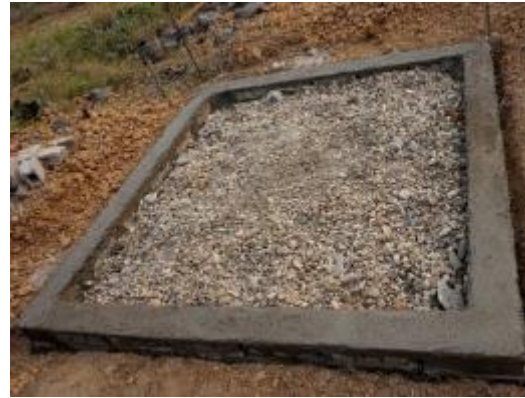
2 Filling gravel in the foundation as a heat barrier
