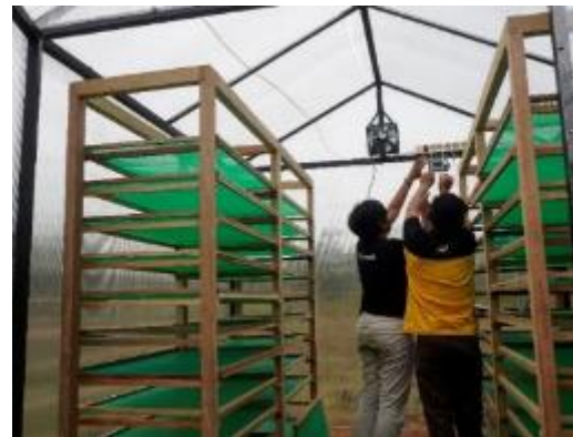
5 Exhaust installation and automatic adjustment system
